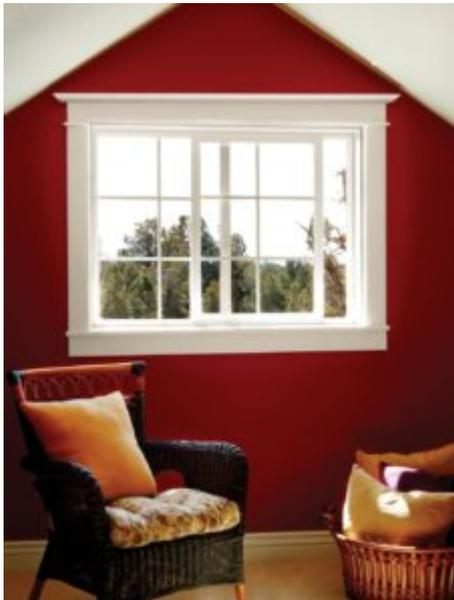
2) These hinged windows operate by a turn of a crank in an operating mechanism. They can be hinged on the left or the right to open outward. Photo courtesy of Marvin Windows
