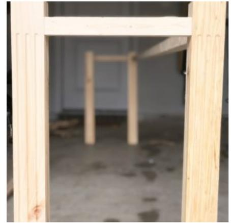
Cut the 2×2's down to 47" and two at 11" for the bottom supports. For this build you can use pocket holes set to a depth of 1-1/2" and pre-drill on the bottom side of the 2×2's. Notice the fluting on the table legs is facing outward. Attach the bottom of the 2×2 supports 2.5" from the bottom of the table leg running even with the start of the fluting. The supports are also centered to allow for 1/2" spacing on each side. Be sure to add wood glue in your joints before attaching the 2-1/2" screws.
